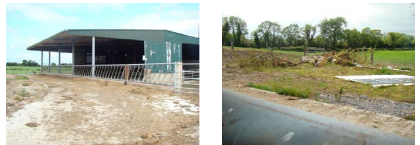
Figure 1: New cubicle house and filled in slurry lagoon
